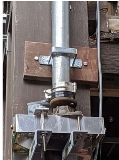
The bearing from an old Water Pump from my "Delica Van" in VK4 served as a rotating base!
