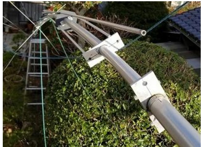
Fig. 2 The 10 m stub popped out from the clamp (view from the end of R9).
